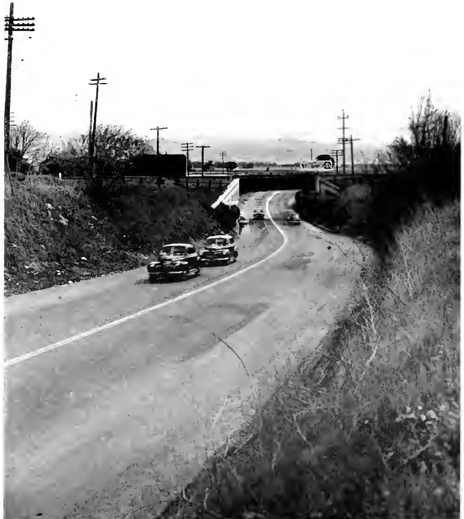
Existing Spence Underpass looking westerly
